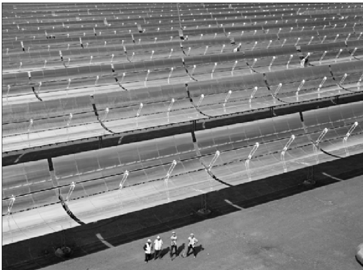
Figure 2 : Centrale Andasol 1, ©Solar Millennium AG.
