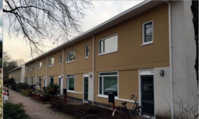
The building blocks of the technical solution for row houses as used in one of the early models. The Energiesprong philosophy does not only apply to external wall insulation. It is about developing industrialized solutions with an energy performance guarantee that are quick to install. This could also include (partial) internal insulation solutions.
