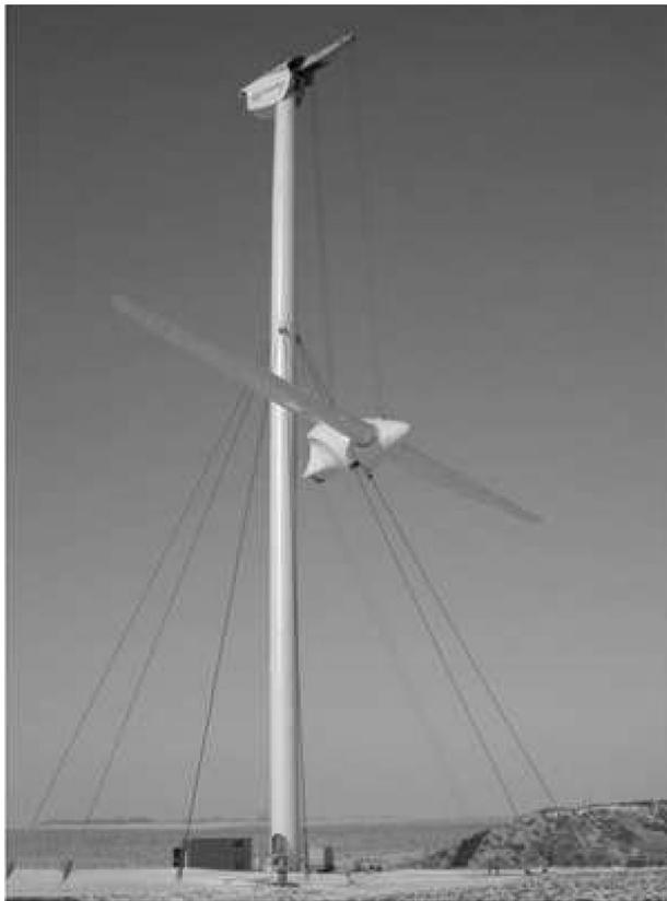
**Photo 5** : Eolienne Vergnet GEV HP 1 MW (Source : Vergnet).
